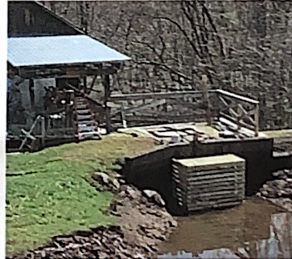
Cage secured in place.
