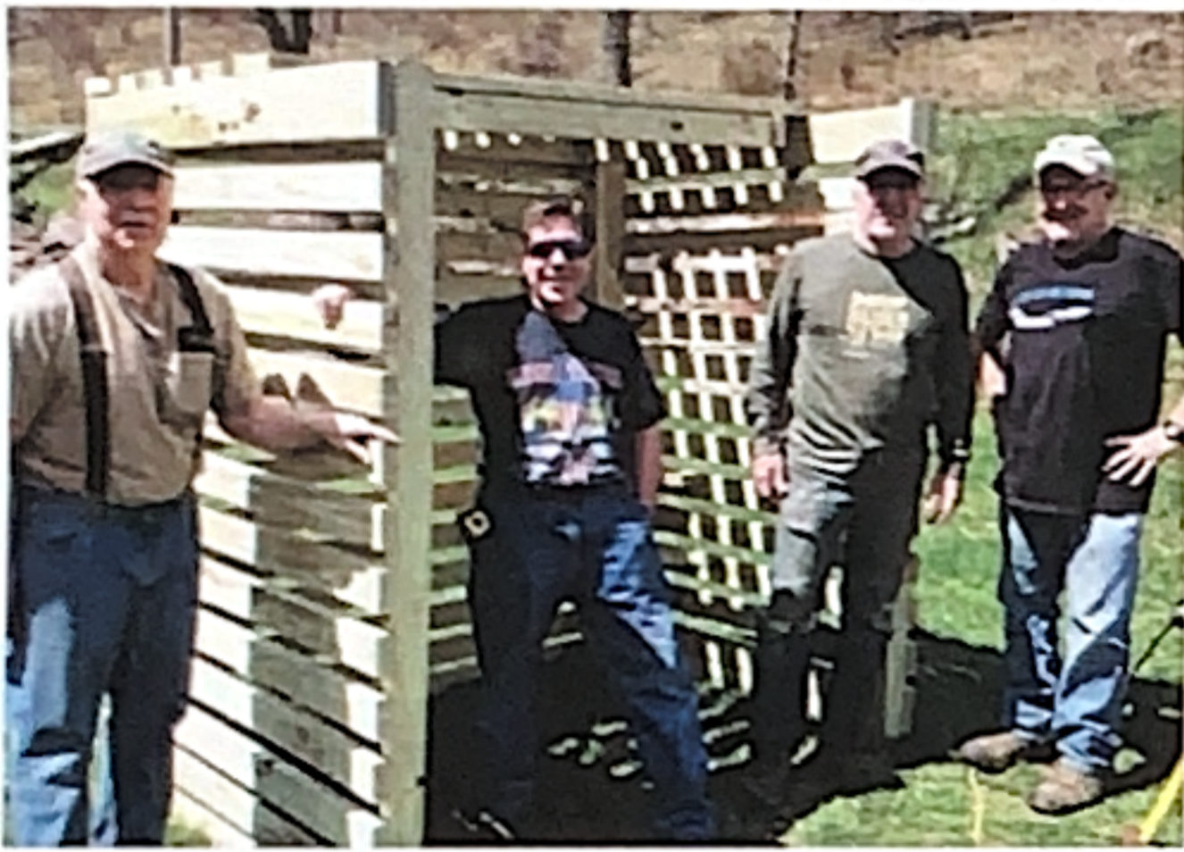
The completed cage ready for installation.
