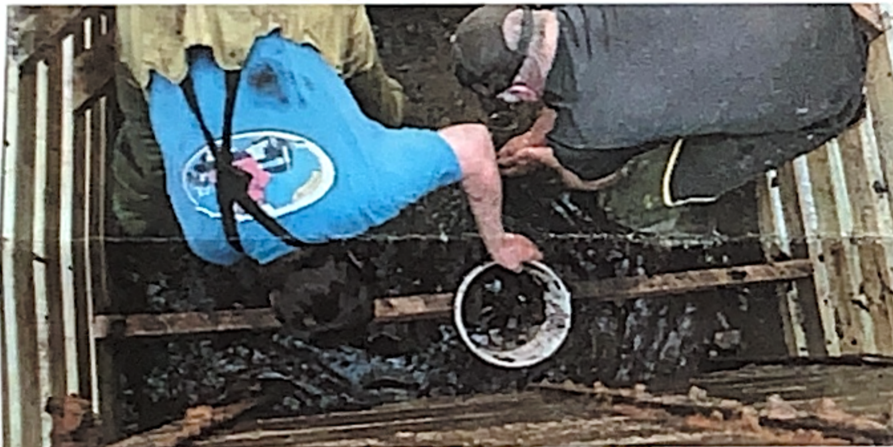
Debris is removed from under the cage and inside.
