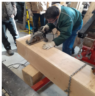
Ron Costantini makes a final cut forming a tenon.
