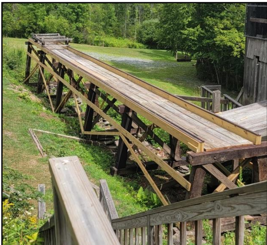
The recently-completed trestle.
