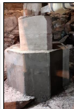
Old pier and stones encapsulated in new concrete.
