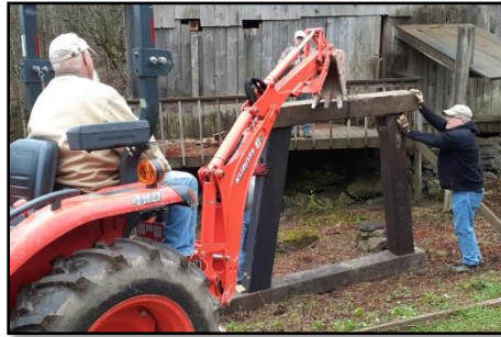
Setting the new railroad tie supports in place.
